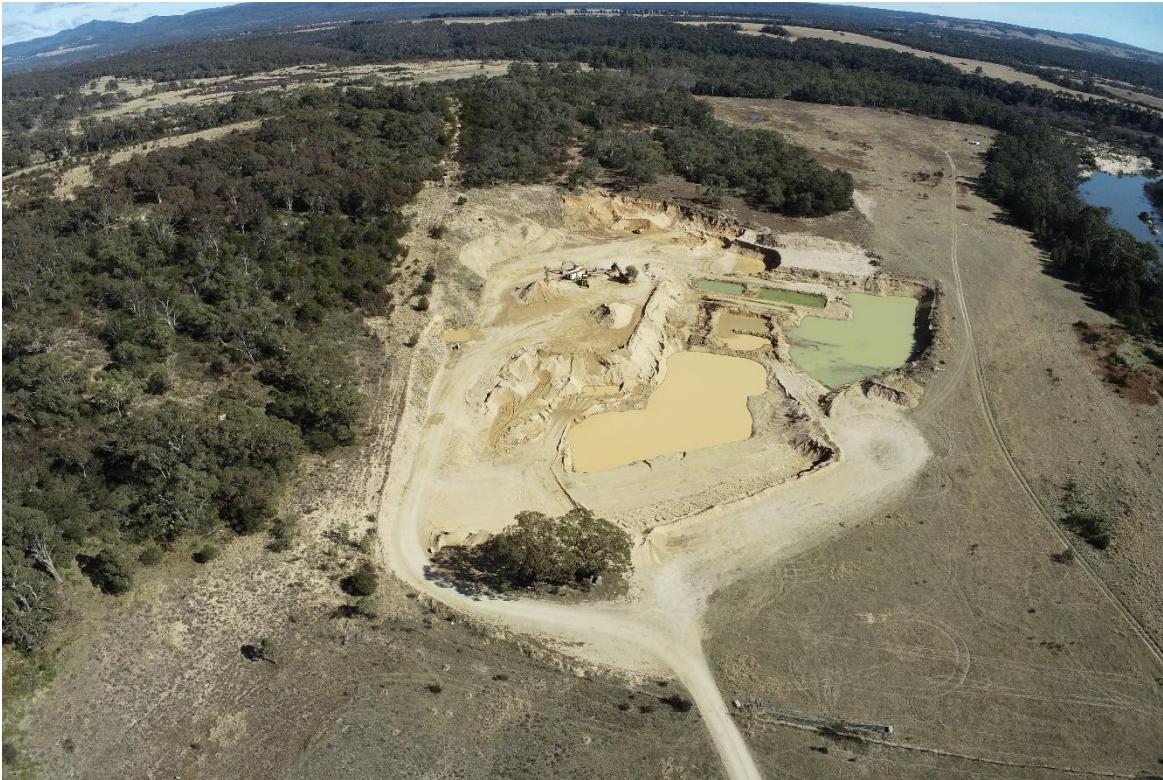
Figure 5.5 Aerial image of current Larbert Quarry operations
